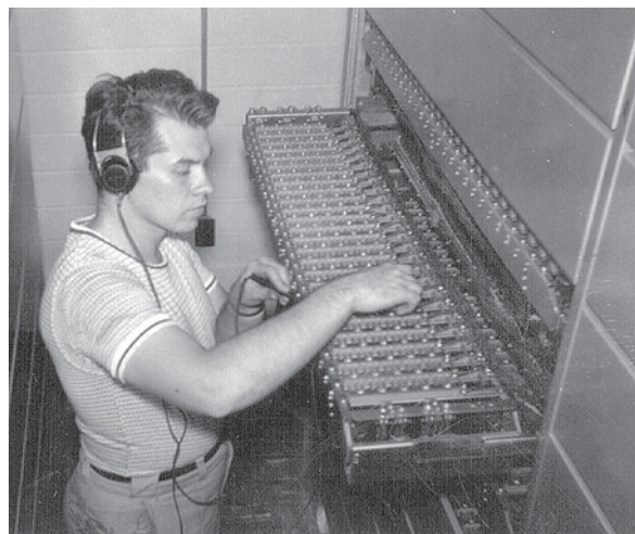
Roger at age 20 testing a Kellogg crossbar switch prior to the cutover of a new 1000 line dial system in Forest City, IA in 1952.
